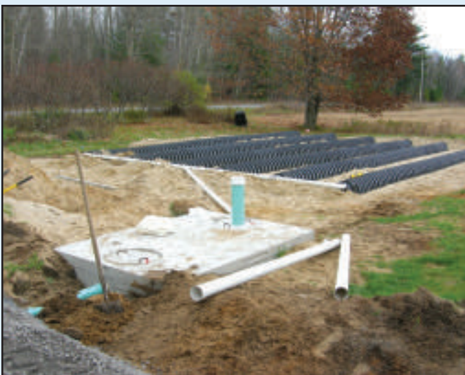
Leaching bed with gravelless trench technology.
