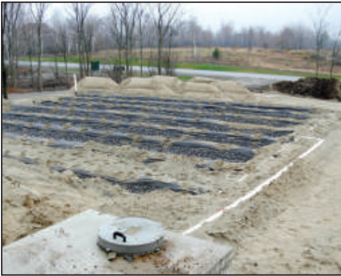
Leaching bed with perforated PVC drain pipes.
