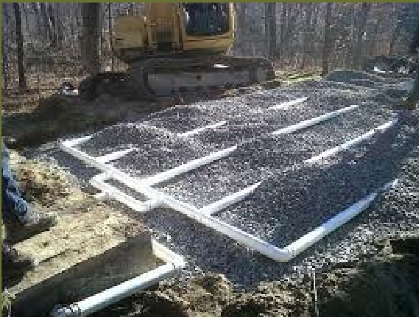
A typical class 4 septic system under construction
